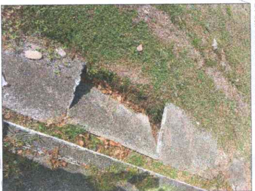
DAMAGE DRAINAGE COVER
